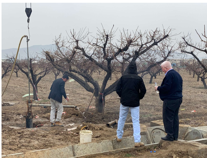
Figure 21. The first gravity fed MAR injection borehole at Badam Bagh in Kabul (Landell Mills, 2019).
