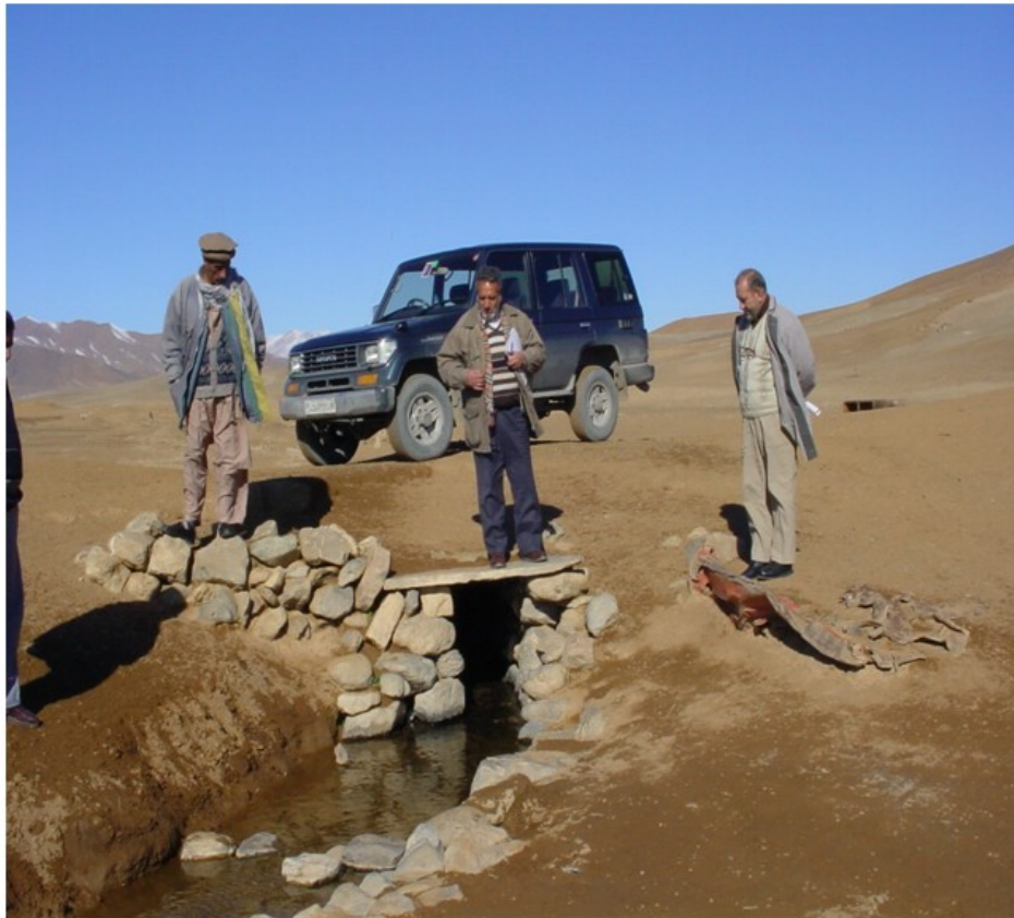
Photo 9: Outlet of a Karez system
