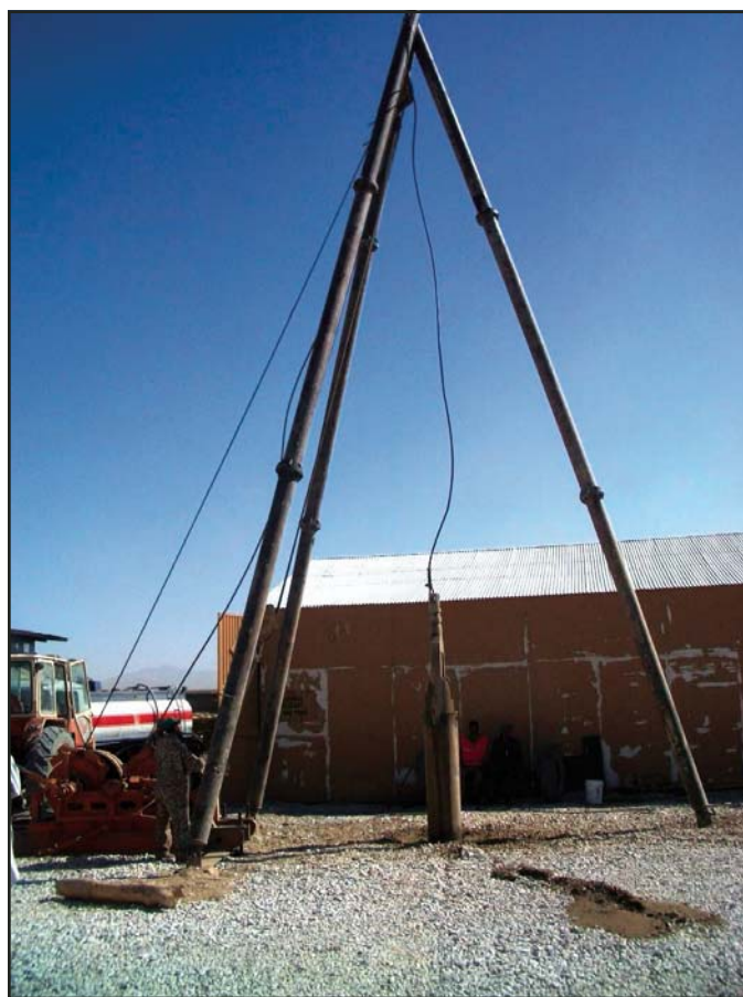
Figure 7. Local Afghan well driller’s “modern drilling machine” during construction of a base camp well.
